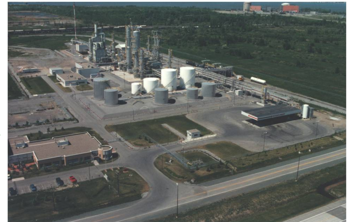
Petresa plant, Bécancour, QC
