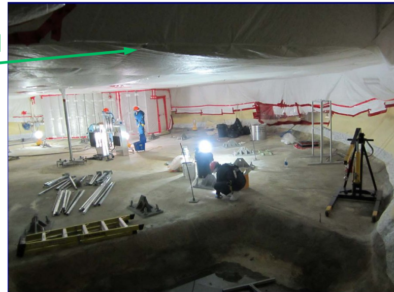
Drilling holes for the anchor bolts
